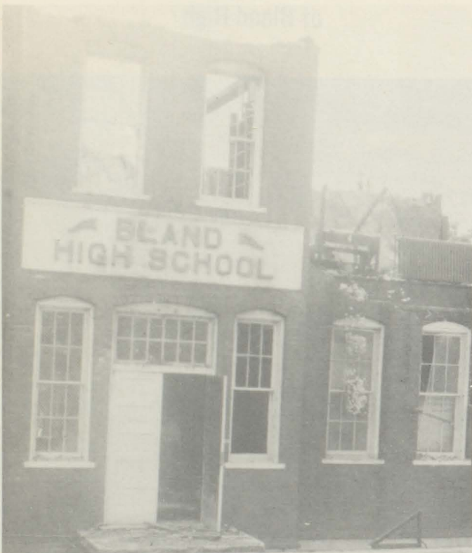
Bland High School destroyed by fire on July 30, 1962.
